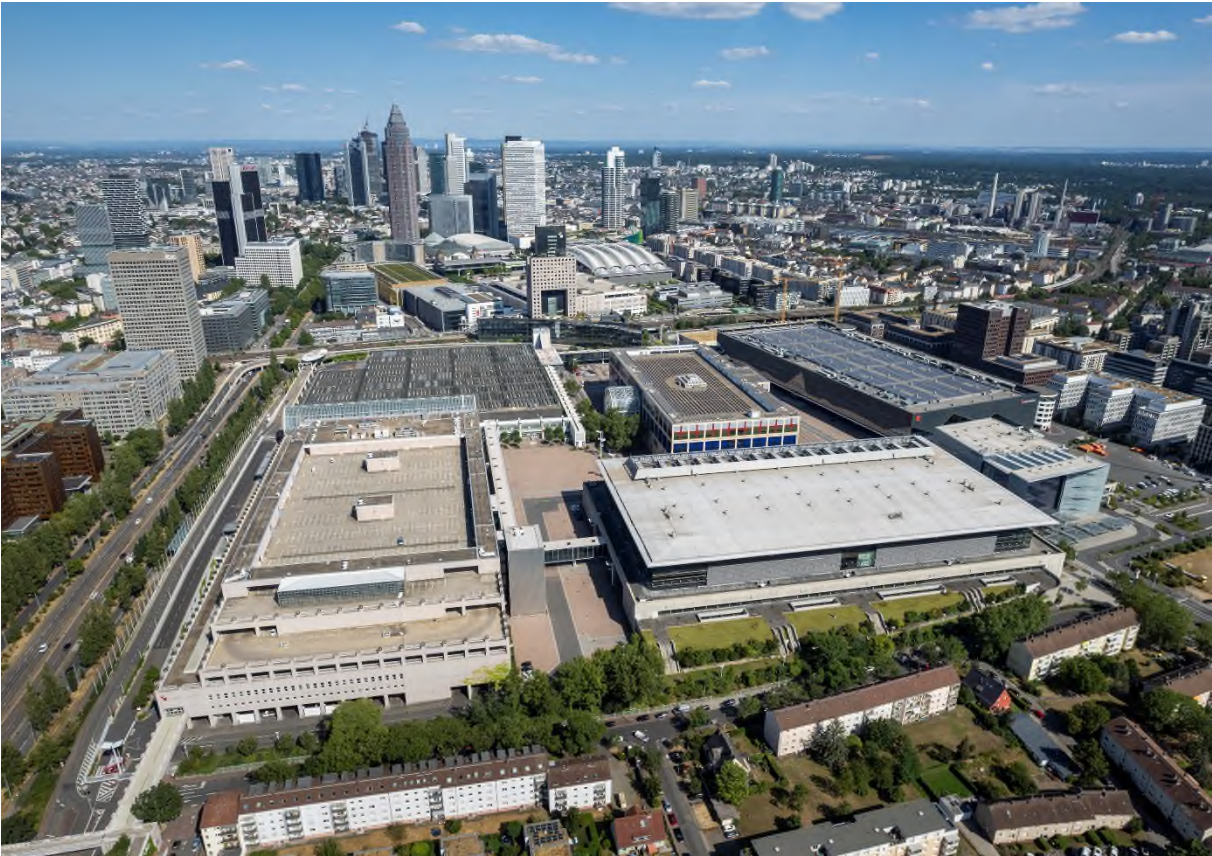
An area of 31,000 square meters of the exhibition grounds is unsealed. In addition, Messe Frankfurt has around 14,000 square meters of near-natural areas designed to promote biodiversity.
